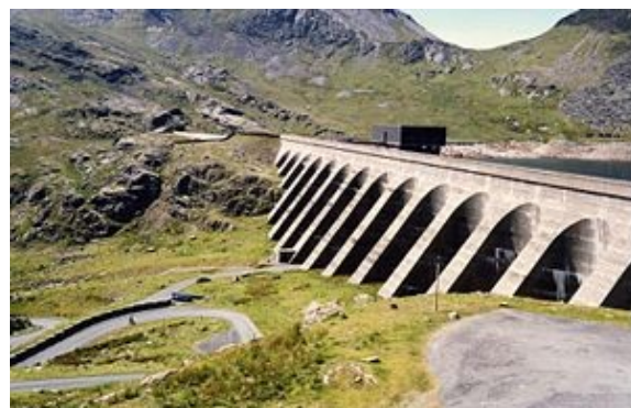
Figure 2 - The upper reservoir (Llyn Stwlan) and dam of the Ffestiniog Pumped Storage Scheme in North Wales. The lower power station has four water turbines, which generate 360 MW of electricity within 60 seconds of the need arising. The size of the dam can be judged from the car parked below.
